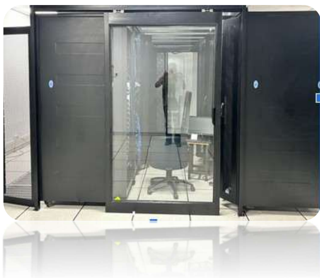
Hot aisle- Containment
